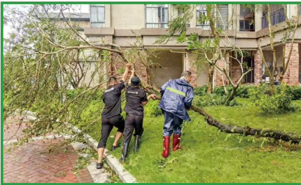
Zhanjiang Branch responded to super typhoon and safeguarded the life and property safety of owners
